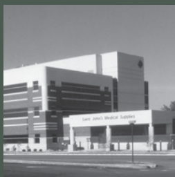
Saint John's Campus Ambulatory Services Center
