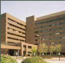
St. Vincent Indianapolis 8402 Harcourt Road
